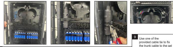
Seperate the gel pieces. Cut cable tie and remove sealing plug from the far left cavity and install the trunk cable. Remove additional plugs and install cables if required. Press the removed gel piece back into place and re-install the gel gland on the HFDC base. Tighten the screw with the recommended torque of 2 N-m.
