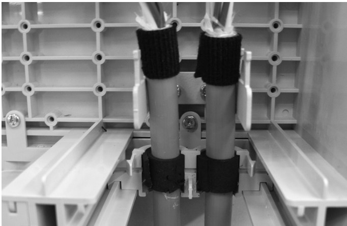
8.11. Position the cable in the box. The foam in the seal area as shown above. For a stubbed cable, use the right port.
