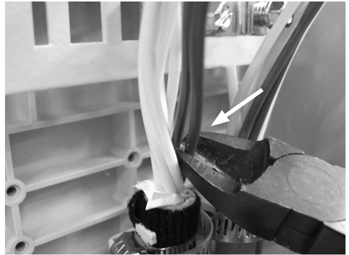
8.16. Cut the required loose tube at the jacket end for a looped cable or take out the required loose tube for a stubbed cable.
