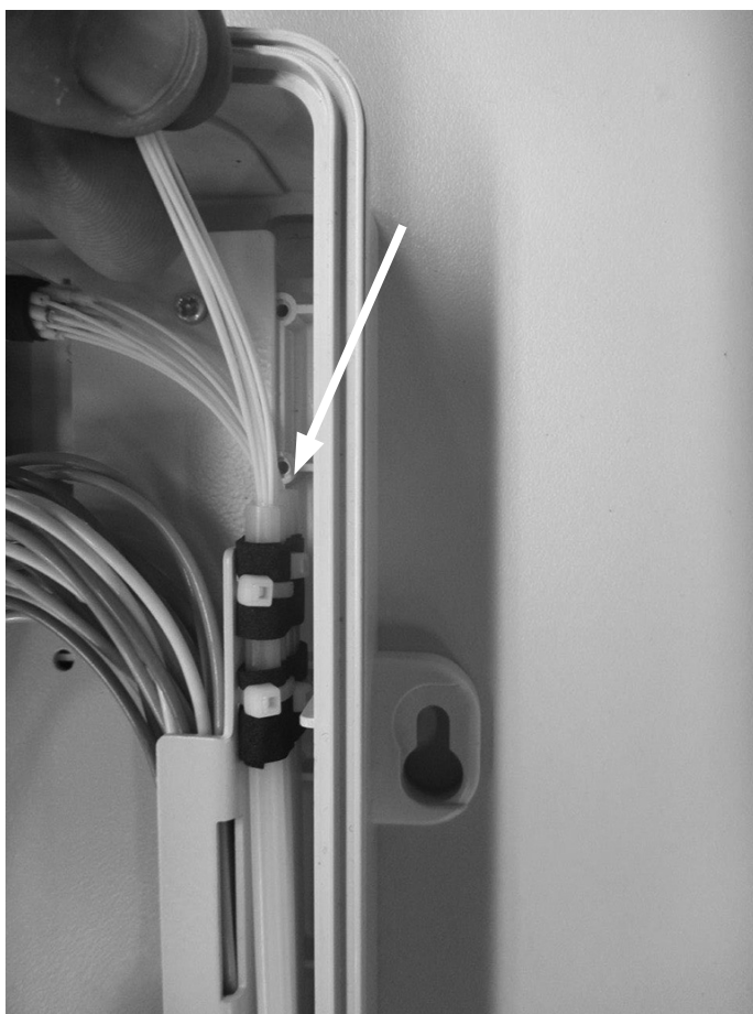
13.12. Route the 900µm fibers to the tray as explained in section 12.8 to 12.11.
