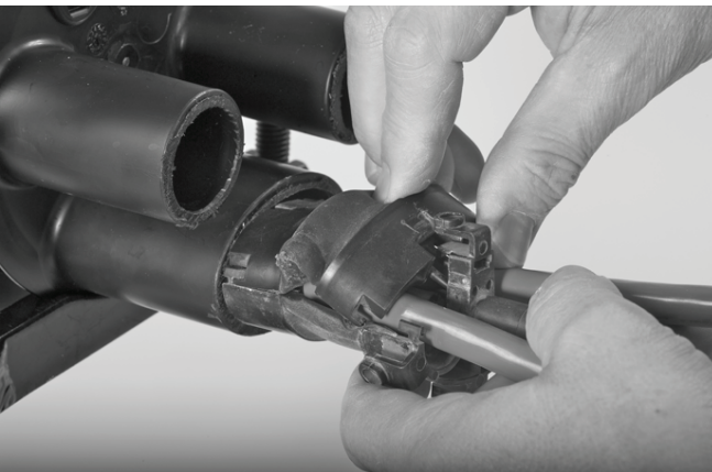
3.2.4 Take the first gel part (with trigger) and put the cables in place, if needed (when large cables) lubricate the cables. Take 2nd gel part and insert the pins in the corresponding holes at top and bottom. Push till snap fit (click).
