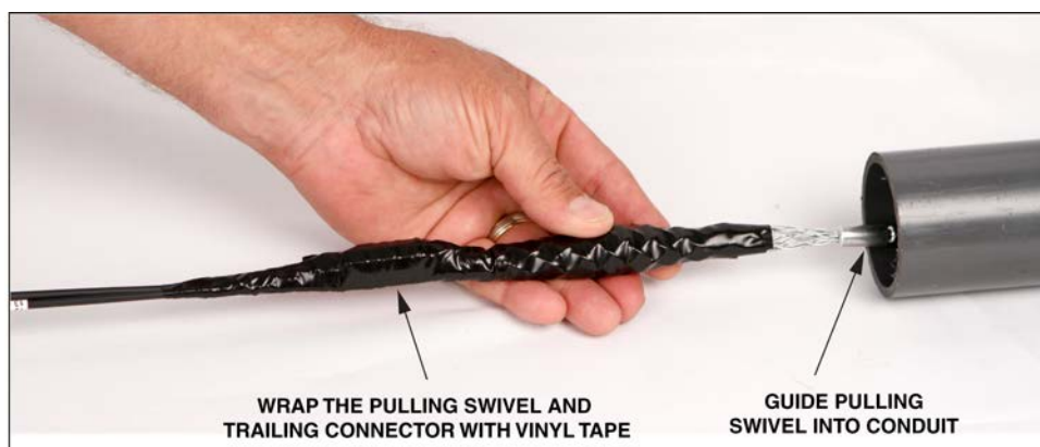
Figure 54. Wrap Pulling Swivel and Connectors with Vinyl Tape
