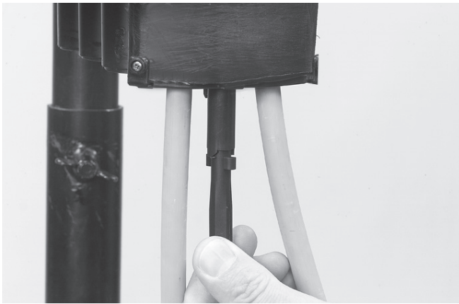
3.2.8 Tighten the trigger till it butts up with the flange.
