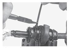
19 Position the 4-out cable separator in between the cables (or plugs), insert in the central part and tighten the tie wraps. Make sure the knobs of the tie wraps are always on top and cut away the tail.
