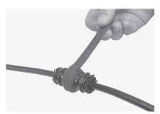
15 Wrap the gel tape around the cable in between the 2 axial pull strips. Note: Do not stretch the gel tape during wrapping. Repeat steps 8 to 15 for all cables.
