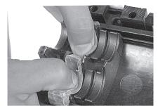
2 Insert the 4 gel profiles in the foreseen cavities at each end of both half shells. Push the profiles to secure in place.
