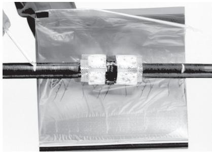
**12.** Centre the sleeve over the adhesive bags and mark the sleeve ends on the cable.
