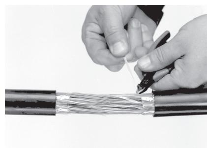
**3.** Remove all unit tapes in the cable opening. Spread the conductors evenly so that there are no groups of conductors tightly bundled. The conductor bundle diameter should be about 5 mm to 10 mm larger than the original cable core diameter.
