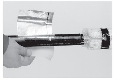
**13.** Wrap the aluminium cable protection foil around the cable, the blue line matching the marks on the cable jacket. Smooth the aluminium foil with a blunt tool.
