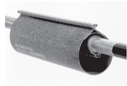
**19.** Immediately align and wrap the second sleeve over the installed and post heated sleeve. Position the channel opposite to the first channel (180°).
