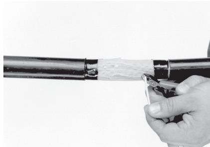
**6.** Insert the channelling pins through the conductors through the conductors at 10 mm from each other. Insert completely and cut-off the excess. Use the left over pieces until the pin is totally used up. Do not force the channelling pin.
