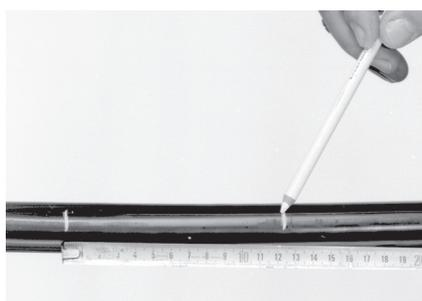
**1.** Using locally approved techniques and tools, remove the cable jacket over a distance of 120 mm.
