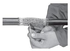
6. Place the channelling pins through the conductors at 10 mm from each other. Insert completely and cut-off the excess. Use the left over pieces until the pin is totally used up. Do not force the channelling pin.
