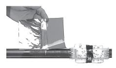
**13.** Apply the adhesive cable wrap with the adhesive portion next to the net tubing. The aluminium part of the cable wrap is positioned a thumb's width from the mark nearer to the adhesive bags. Smooth the aluminium foil with a blunt tool.
