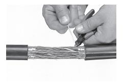
4. Remove all unit tapes in the cable opening. Spread the conductors evenly so that there are no groups of conductors tightly bundled. The conductor bundle diameter should be about 5 mm to 10 mm larger than the original cable core diameter.
