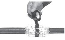
**11.** Wrap the adhesive bags around the cable opening, mesh side down. Secure in the middle with PVC-tape.
