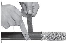
9. Abrade the cable circumferentially over the cleaned distance.
