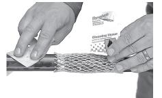
8. Remove the cleaning tissue from its packaging and clean the cable jacket on both sides of the cable opening over a distance of 100 mm.
