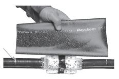
**12.** Centre the shortest tubular sleeve over the adhesive bags and mark the tube ends on the cable.
