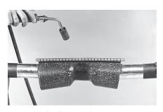
16 Center the sleeve and start recovering it in the middle on the opposite side of channel. Heat until the paint changes colour from green colour to black.
