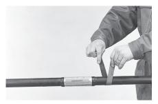
8 Abrade the cleaned area of the cable circumferentially. Remove abrasion dust with a clean, dry cloth.
