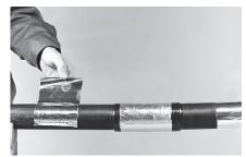
11 Apply aluminium foil on the cable jacket from inner mark, away from splice. On lead cables the aluminium foil is not needed.
