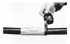
**6** Tape, the liner down onto the cable on both ends. Tape maximum 5 mm on the cable to avoid shortening of the bondlength.
