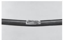
2 Select the appropriate kit according the distorted area and trouble bundle. Trim away the PE-sheath of the cable, respecting the maximum recommended opening. Repair damaged conductors with local approved method. If complete removal of jackets is needed, repair earthing of cable.
