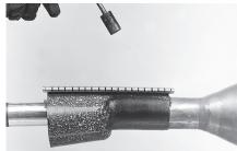
17 Recover the sleeve up to the end, moving the flame circumferentially until the paint has changed colour from green to black. Apply extra heat to the end of the sleeve around the cable end for about 30 seconds.
