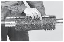
14 Install the heat-shrinkable wraparound sleeve around the splice. Pull the channel over the rails.
