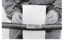
**5** Install the liner around the cable opening such that the middle of the finer matches the middle of the splice. Wrap tightly around the cable and smooth alu-liner; cut it to size such that there is a 40 mm overlap.
