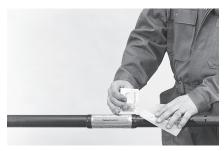
7 Clean the entire circumference of the cable jacket over a length of 200 mm on each side of the liner. Use a cleaning tissue supplied in the kit.
