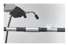
13 Flame brush the entire cable surface to be covered by sleeve for about 10 seconds on each side of the splice. For lead cables preheat the lead up to  $\pm60^{\circ}$ C (hot to the touch).
