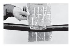
**3** Take alu-liner and preposition it according to the cable direction as indicated on label.
