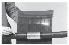
**9** Position the heat-shrinkable sleeve over the splice so that it covers the cables on an equal distance. Mark the ends of the sleeve on the cable jacket.
