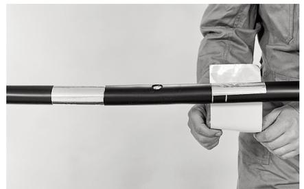
**6** Apply aluminium foil on the cable jacket, away from the hole starting from the inner mark.
