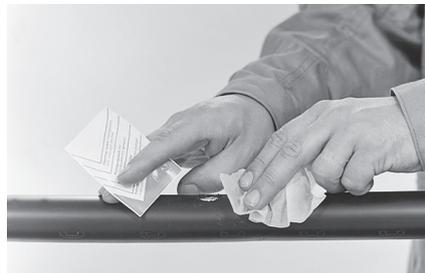
**2** Clean the entire circumference of the cable jacket over the whole sleeve length with the cleaning tissue supplied in the kit.
