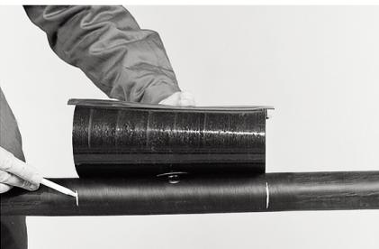
**4** Position valve over hole and mark ends of sleeve on cable jacket.
