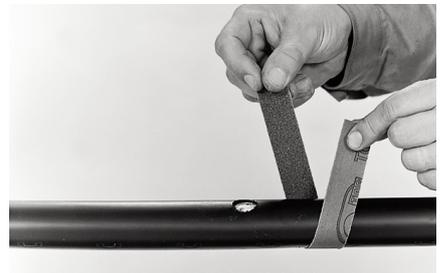
**3** With the abrasive strip supplied in the kit, abrade the cable circumferentially over the entire cleaned length. Remove the abrasion dust with a clean, dry cloth.
