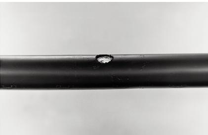
**1** With a locally approved tool (e.g. hot knife), make an 18 mm diameter hole in the cable jacket and the metal screen where the valve is to be inserted. Be careful not to damage the conductors.
