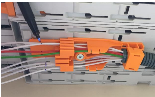
4.1.1 Mark the stripping point on the loose-tubes make sure that there is an overlap of 1cm behind the fopt-holder
