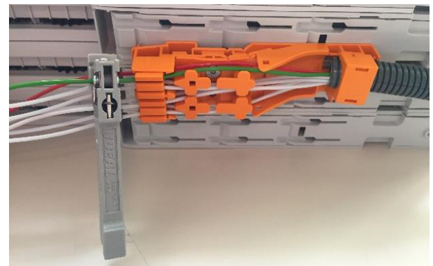
4.1.2 Cut the loose-tube at the marked point and clean the fibers
