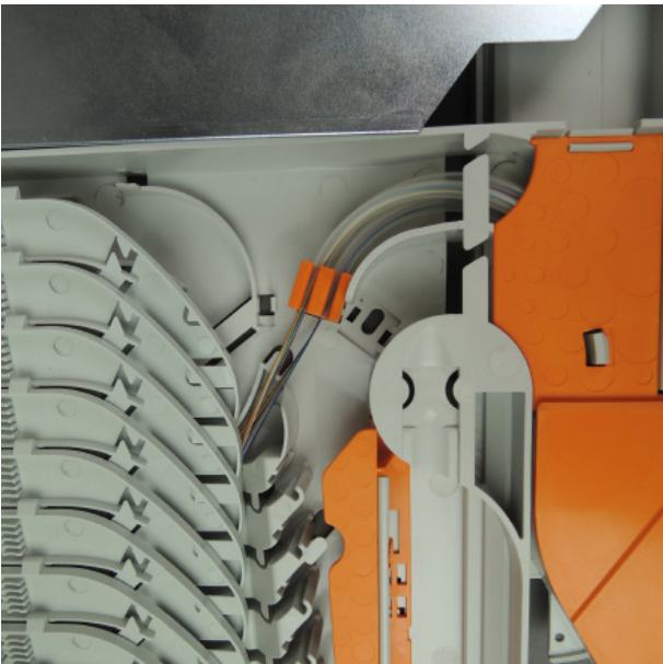
3.2.3 Click the fopt-holder(s) into the splice drawer and guide the fopt-tubes as shown in the picture
