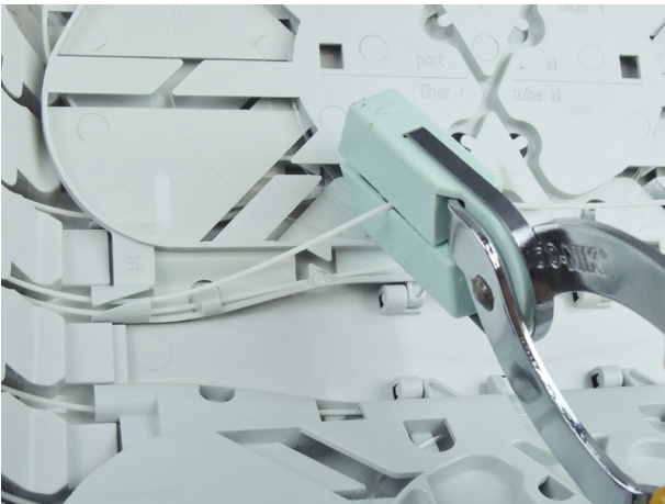
3.9 Strip the 900 \mu m to 250 \mu m with a proper tool
