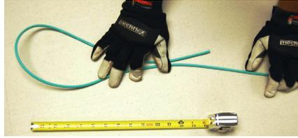
2. Holding the loop, twist the cable three or four times. Using electrical tape, securely wrap the cable going all the way up to the loop and then all the way back down.
