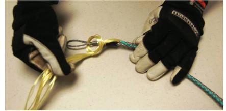
5. Slide the cable back into the mesh grip until the aramid is taught. Wrap the aramid yarn tail around the mesh grip. Using electrical tape, cover the aramid to protect it during the pulling process. Also tape the mesh grip to the cable jacket at the entry point.
