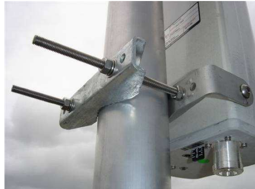
Figure 1: Correctly Assembled Mounting Bracket for Fixed Downtilt Antenna
