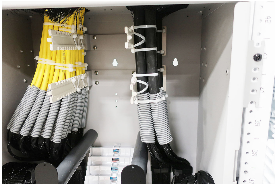
Figure 20. Example of Facility Cable Clamping
