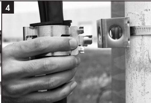
Insert SnapStak hanger into 3/4" mounting hole adapter or cable ladder. SnapStak hangers can be stacked 2 high maximum.
