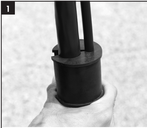
Insert cables into grommet.
