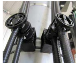
Hangers Installed with SA-1C
