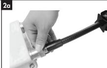
Connect the 1/2" connector to the device port and hand tighten. Device port must be free of tar, butyl, and vinly tape residue before beginning this step.
