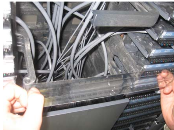
Figure 2. Vertical Trough Hole Alignment/Spacing
