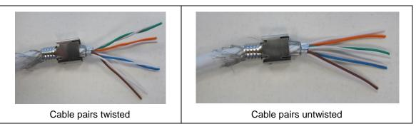
Figure 4. Untwist Cable Pairs
